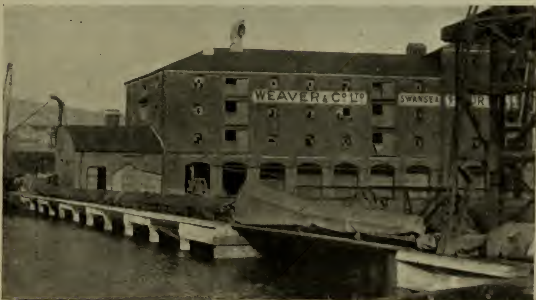
NEW QUAY AT SWANSEA.
